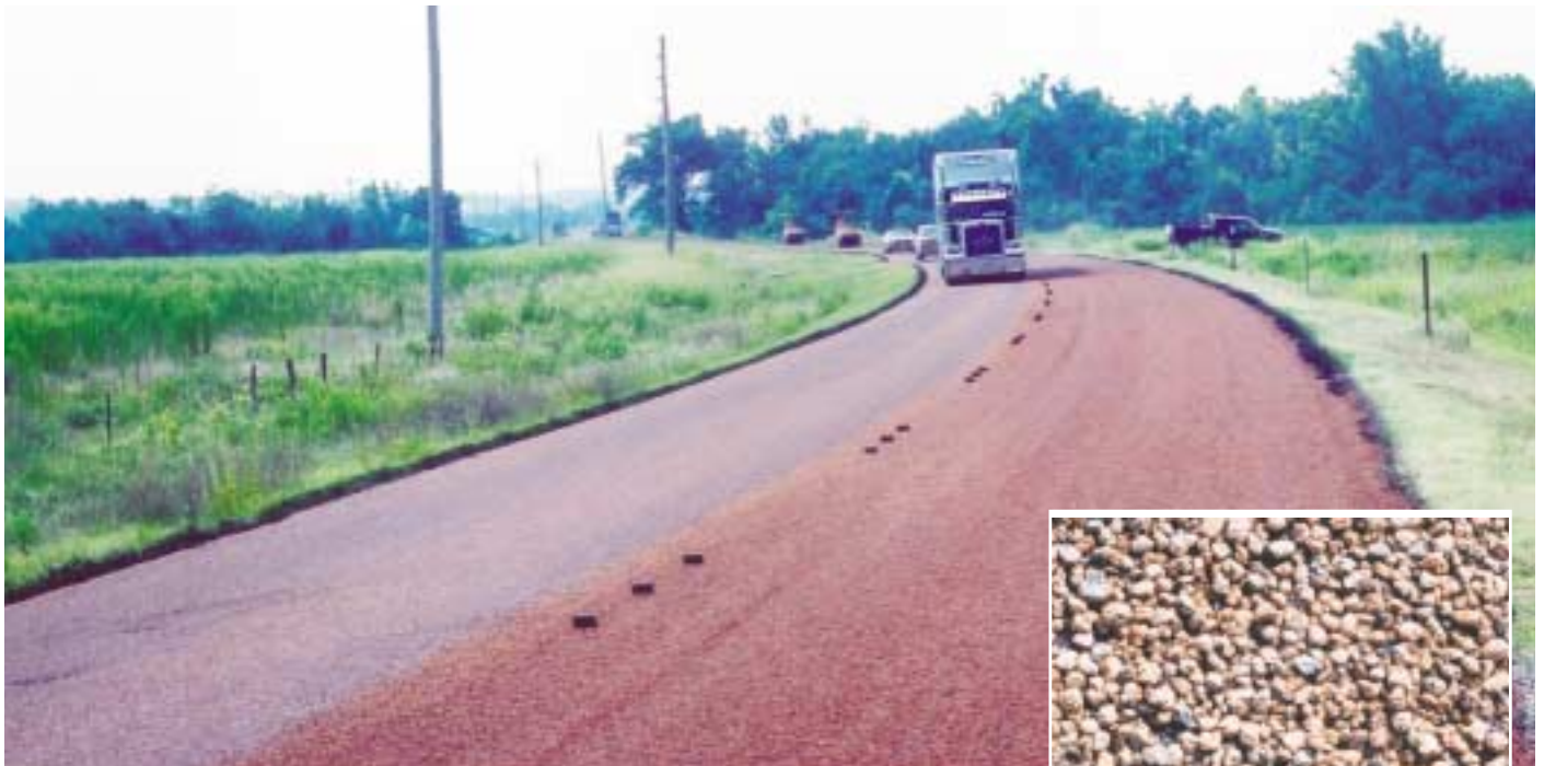
Traffic following a flag car on the left. Road on right has been rolled and broomed, is two-hours old, and about ready for traffic. (Inset) a close up one-hour old.
